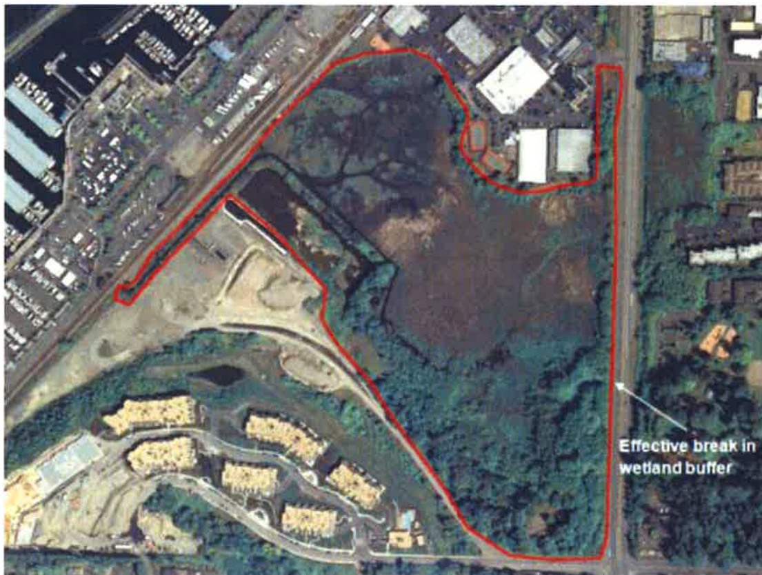
Figure 2. Edmonds Marsh and Willow Creek west of SR 104 with intact buffers outlined in red. Note tidal channels draining the western portion of the marsh.
